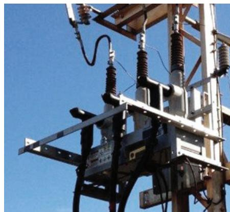
Figure 11: Elbow-Connected G&W Viper Reclosers
